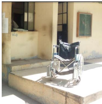
At Main Security Office
